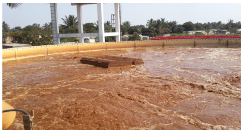
Figura 13: Reactor Sequencial Biológico
