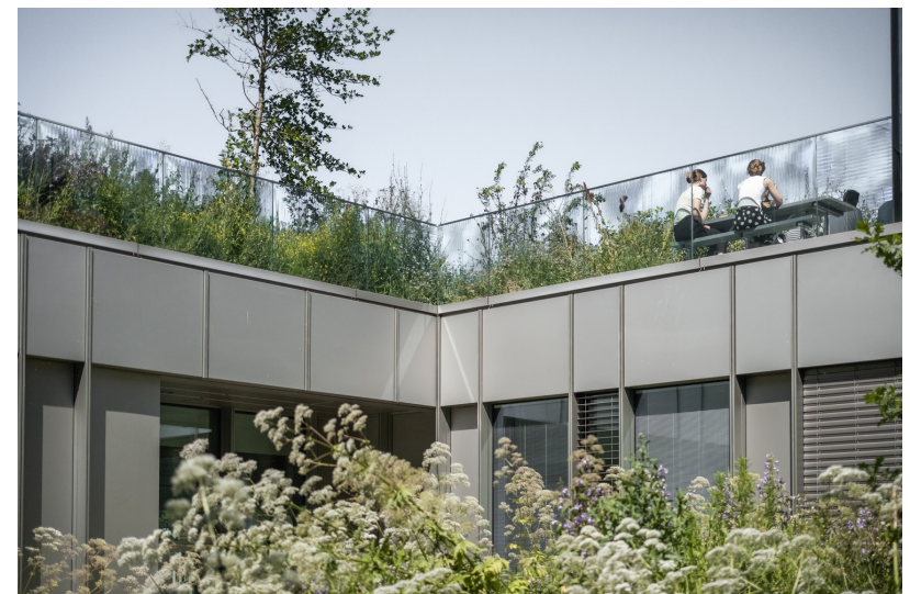
Figura 38 - Steno Diabetes Center. Fonte: https://www.archdaily.com/1006085/steno-diabetes-center-copenhagen-vilhelm-lauritzen-architects-plus-mikkelsen-architects-plus-sted?ad_medium=gallery
